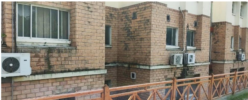
Energy efficient inverters (Combined Cooling Heating and Power Integration Unit)
